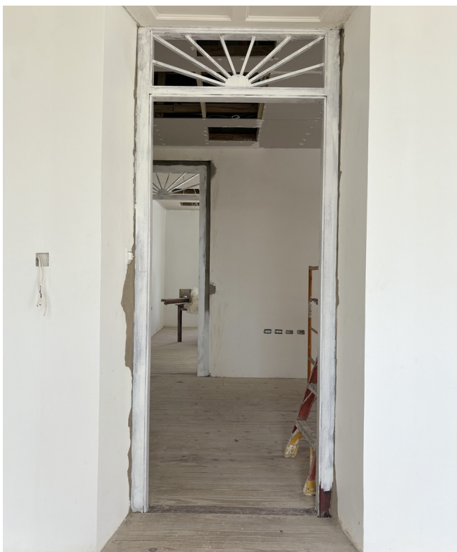
Priming of the main office's doorframes.
