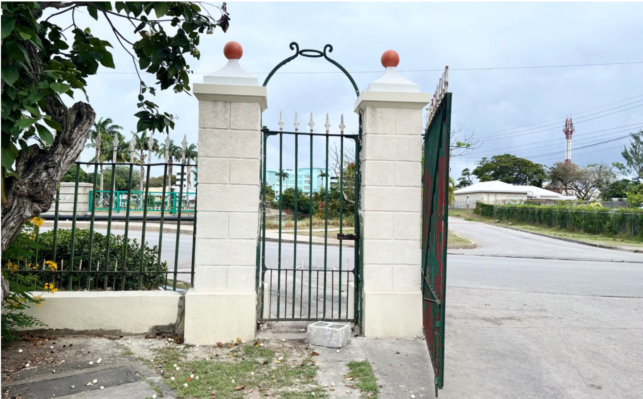
A view of the coral rendered columns at the President's gate in Queen's Park.
