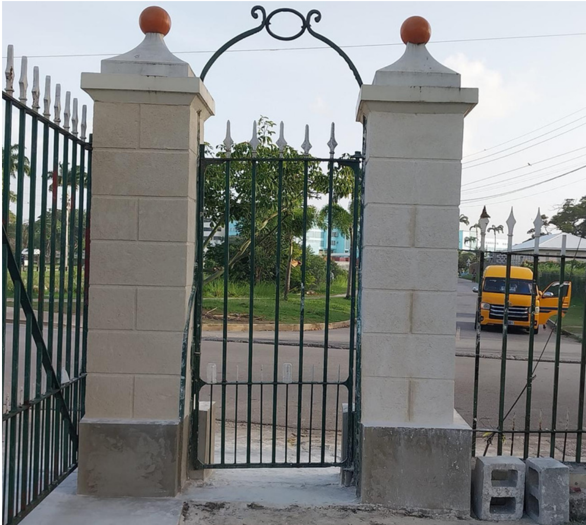
Partial completion of the columns at the President's gate.
