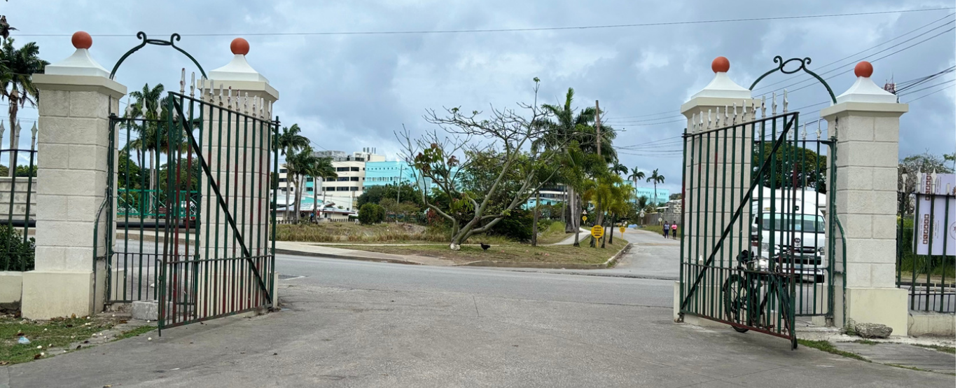
Full view of the coral rendered columns at the President's gate in Queen's Park.
