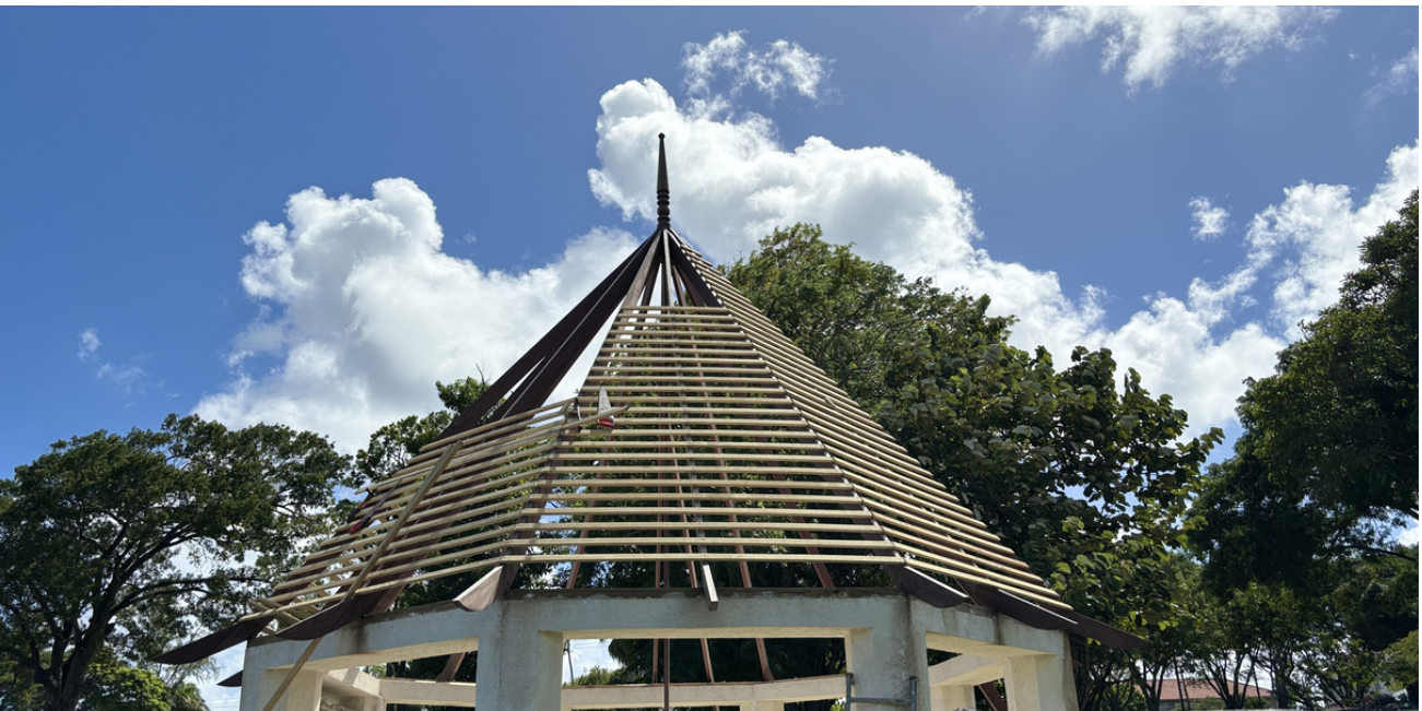
The Trash House's roof - November, 2023
