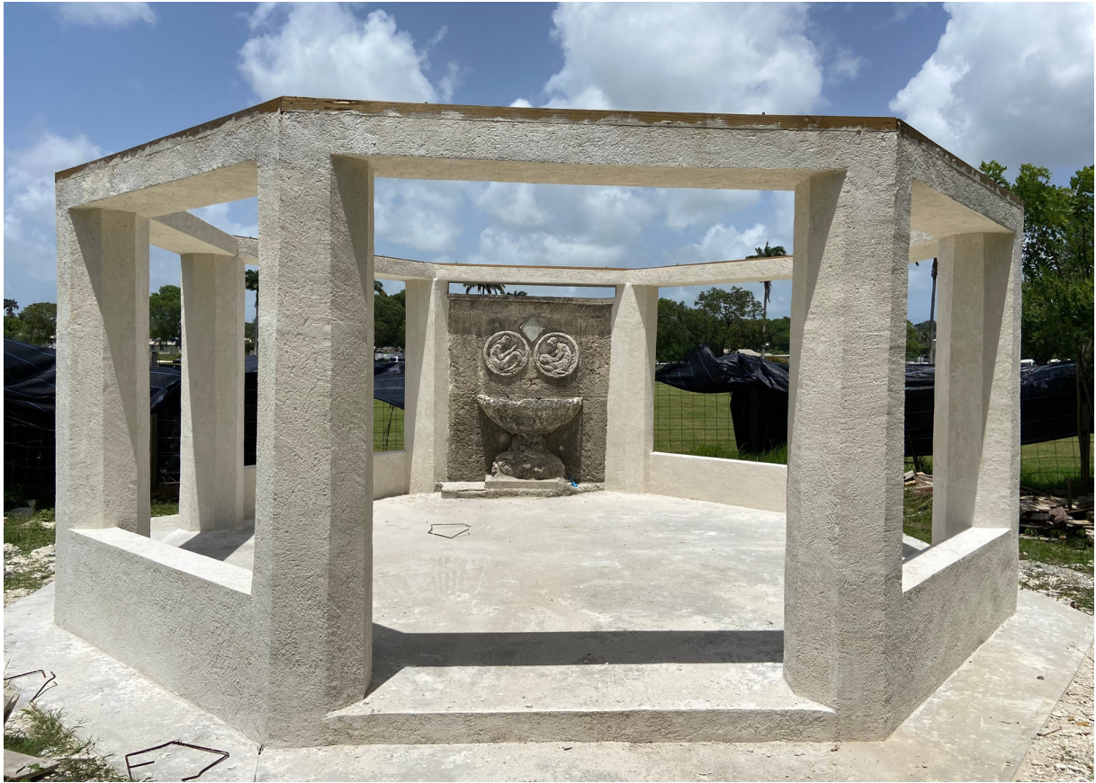
The Trash House in Queen's Park - August, 2023
