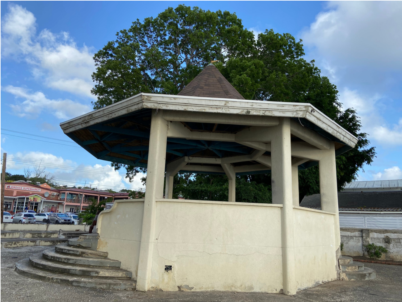
Side view of the Fitts Village Gazebo in July, 2022.
