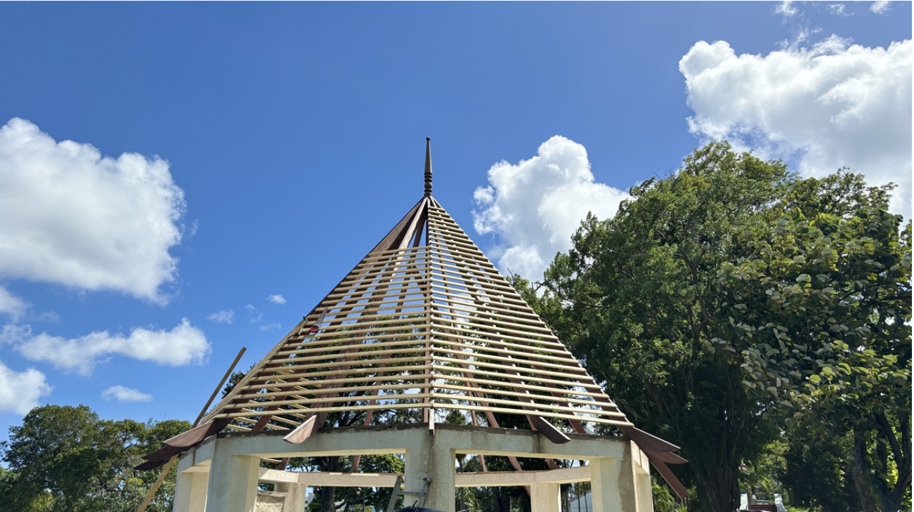
The Trash House's roof - November, 2023
