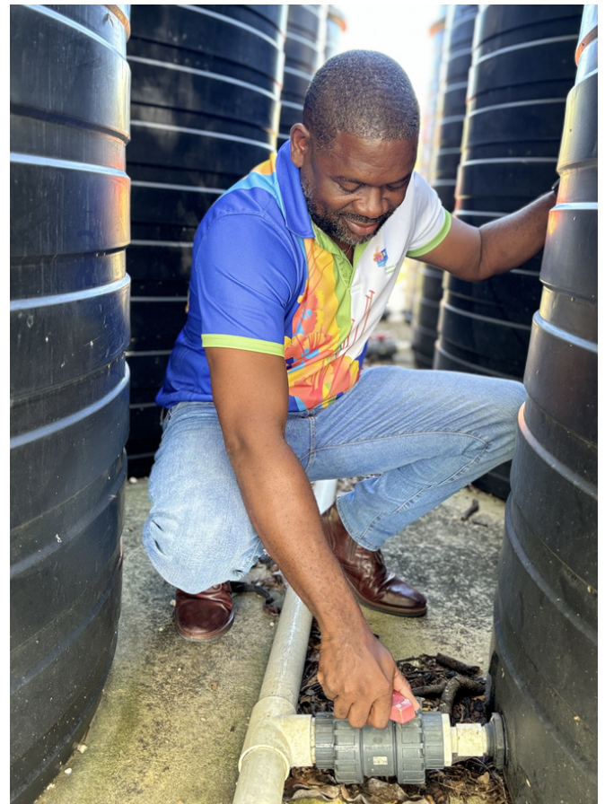
NCC's Senior Electrician, William Husbands.
