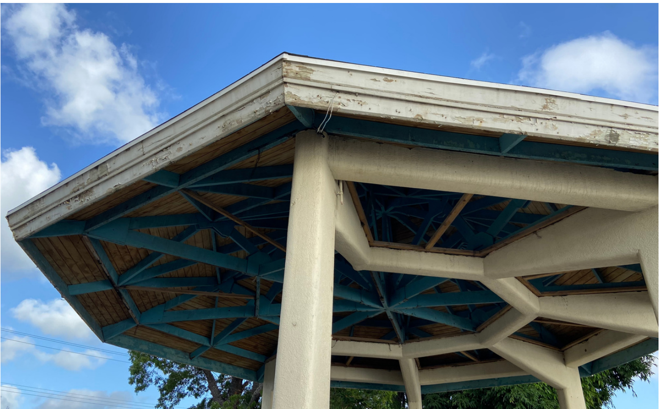
Side and partial back view of the Gazebo's roof in July, 2022.
