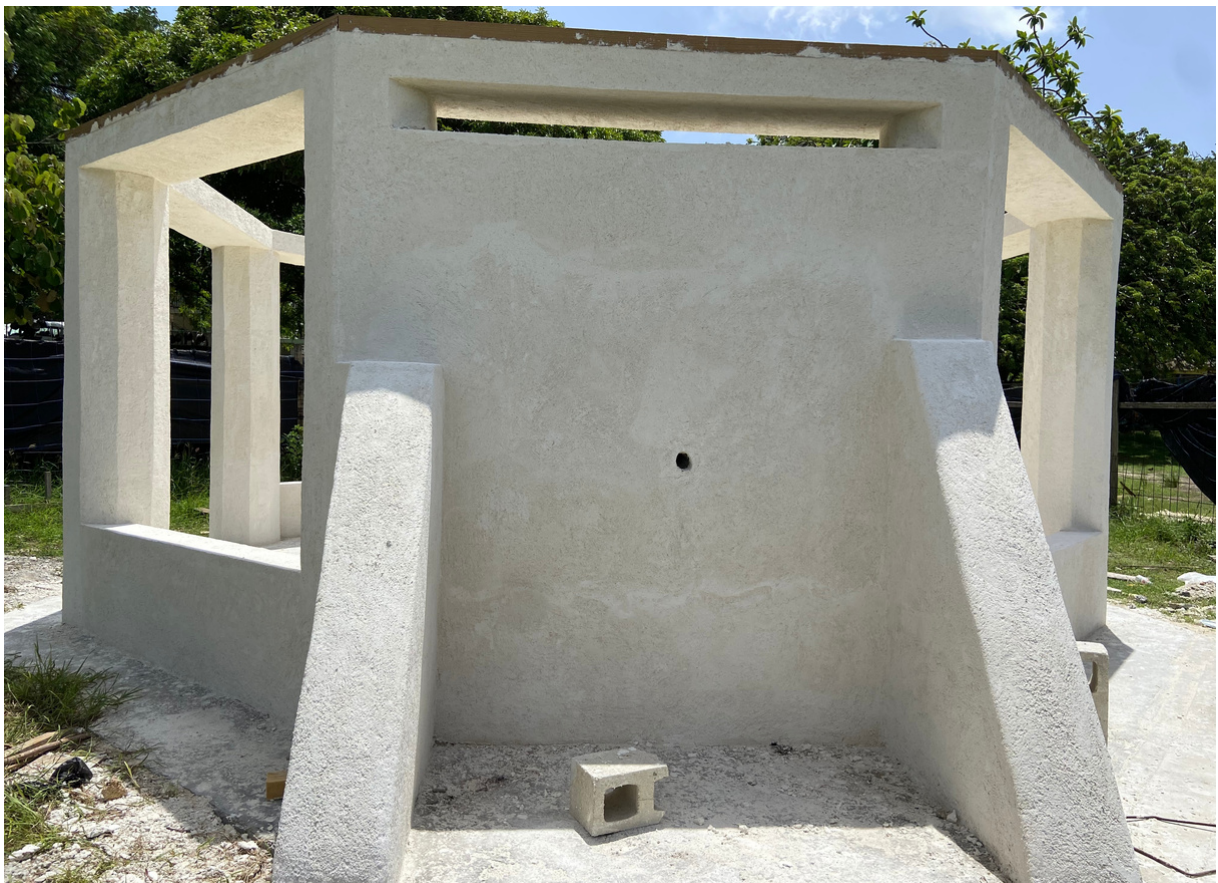
The Trash House in Queen's Park - August, 2023
