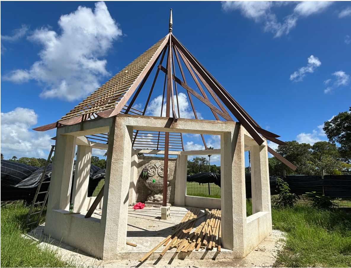
The Trash House in Queen's Park is under construction.
