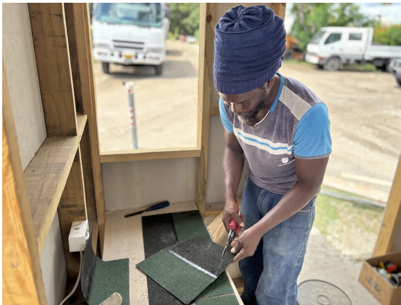
Artisan, Junior Sealy, cutting the materials for the shingles application on the roof.
