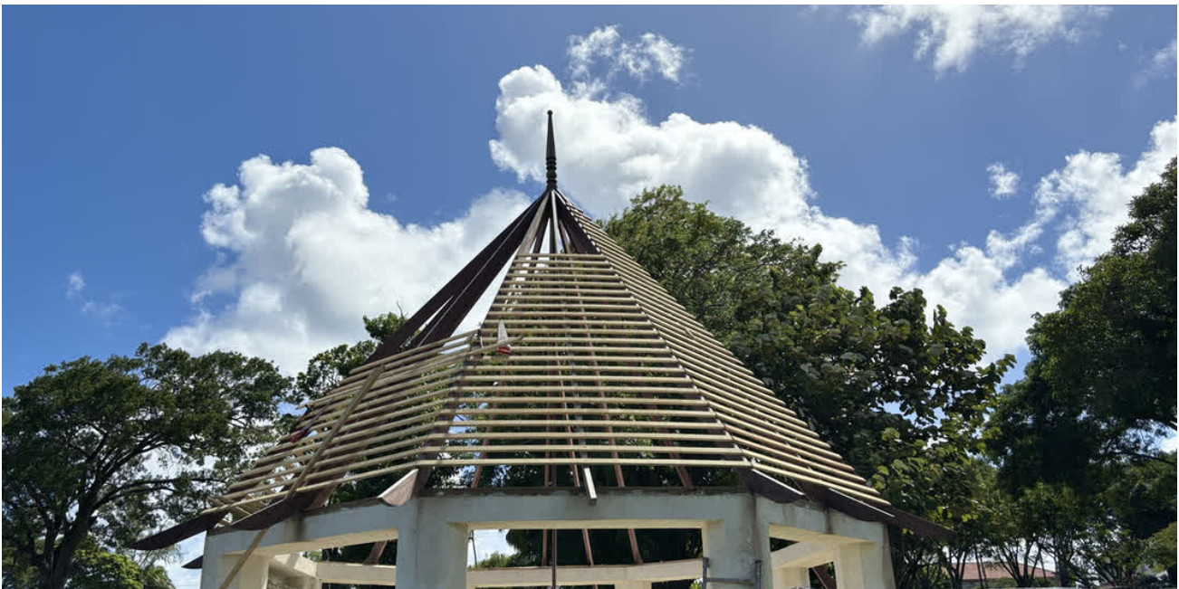
The Trash House's roof - November, 2023
