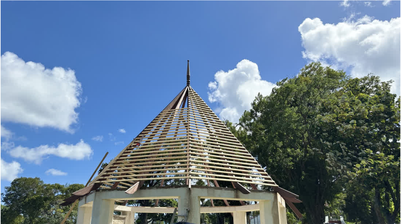
The Trash House's roof - November, 2023
