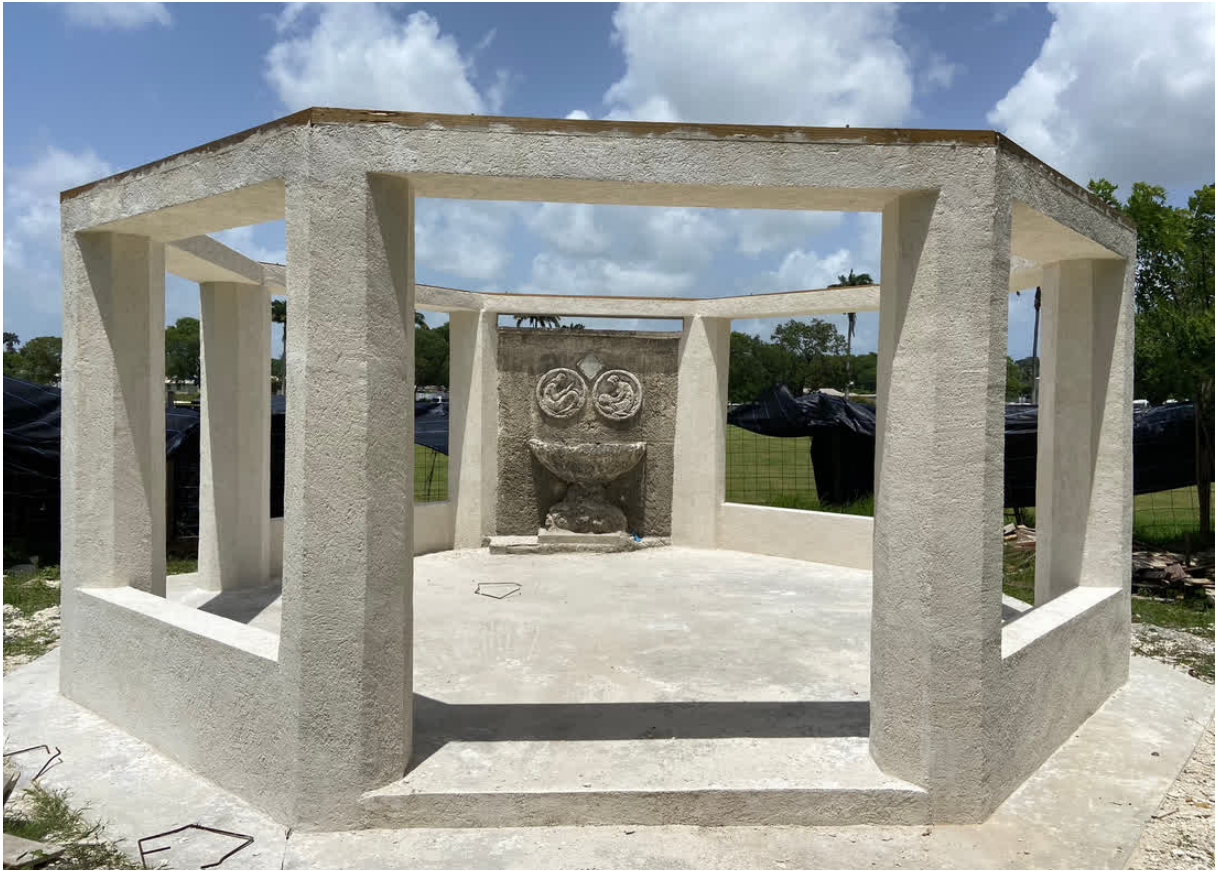
The Trash House in Queen's Park - August, 2023
