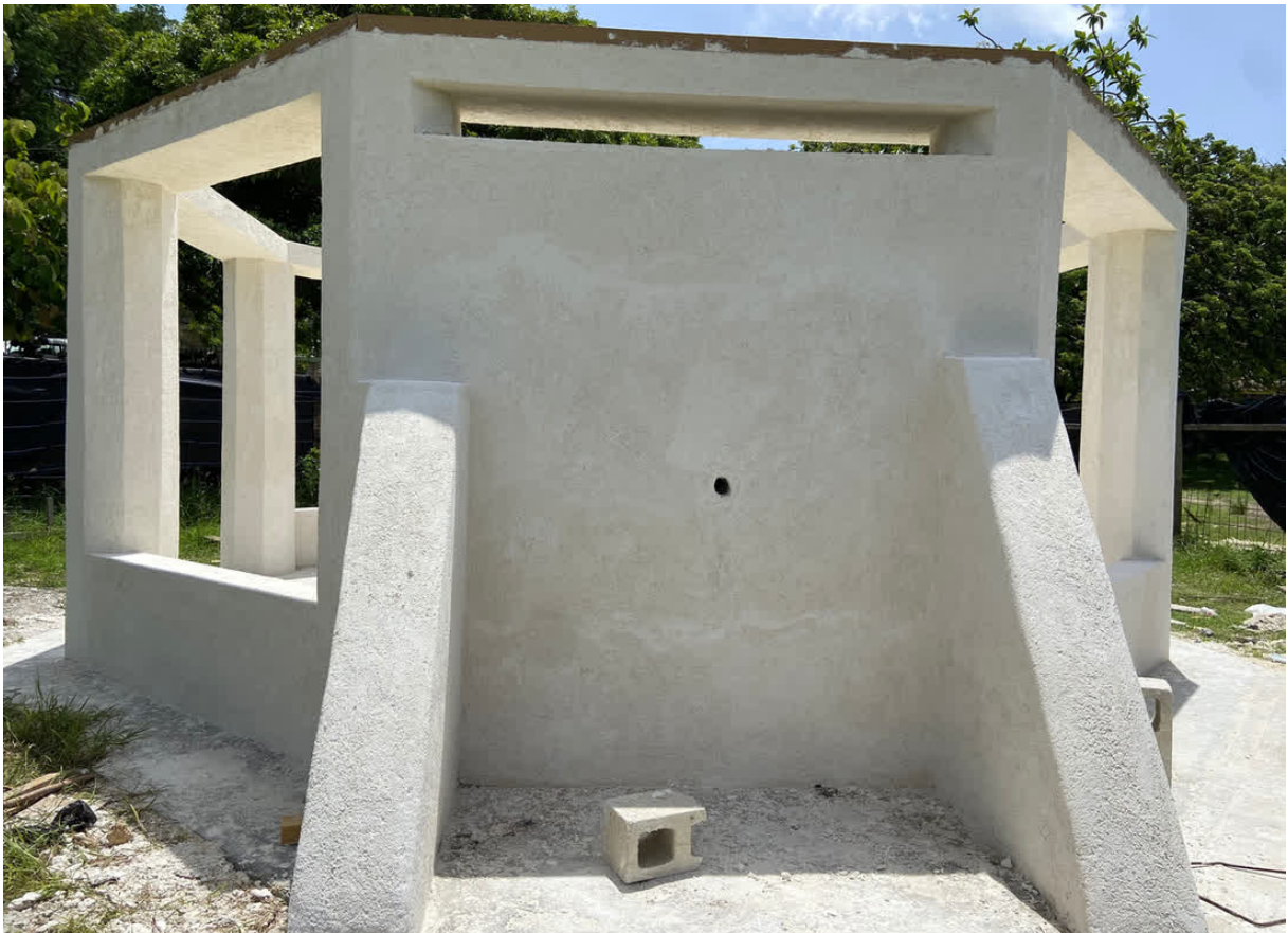
The Trash House in Queen's Park - August, 2023
