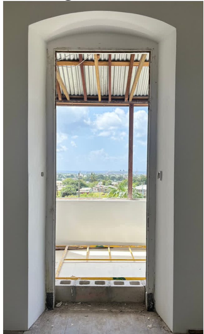
An access point to the building's balcony.
