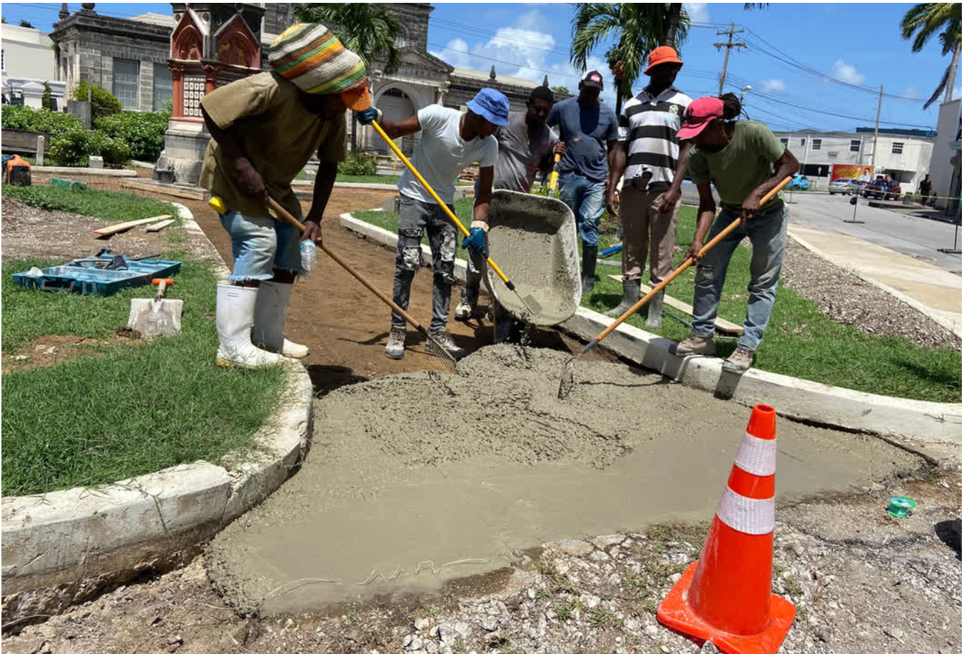
All hands were on deck as the artisans continued to pour and spread the concrete.
