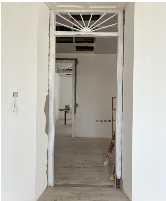
Priming of the main office's doorframes.
