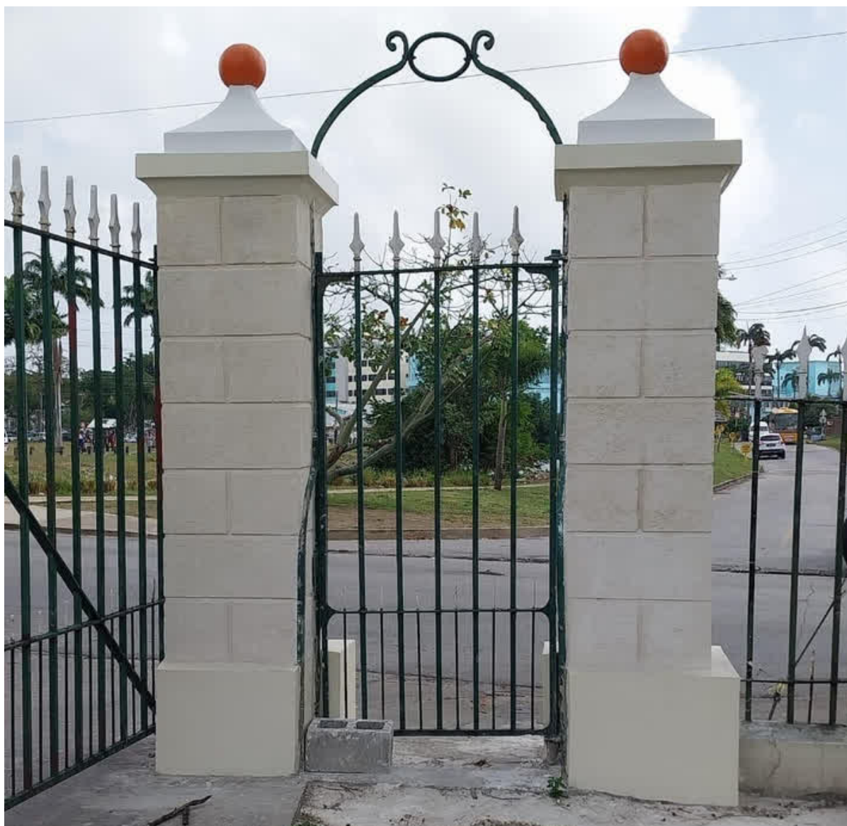
A closer view of the coral rendered columns at the President's gate.
