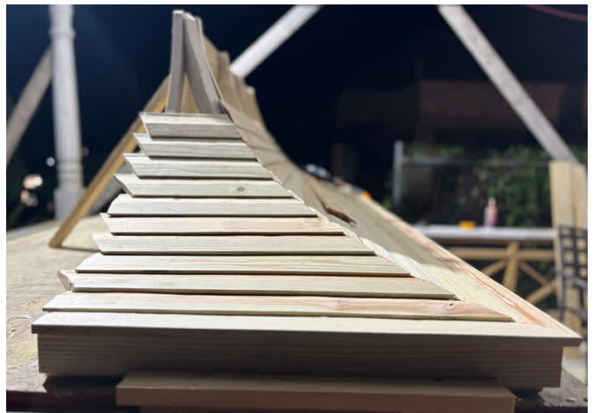
The stacked pattern of the hood with various lengths of timber for the shape.
