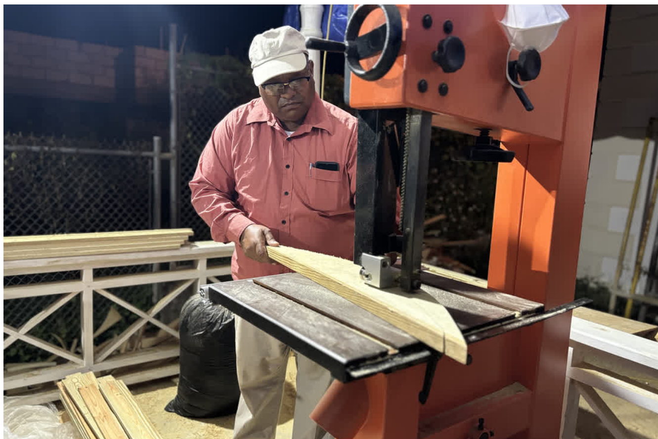
Bhopal Sundar carefully cutting a piece of timber for the window hoods' design.
