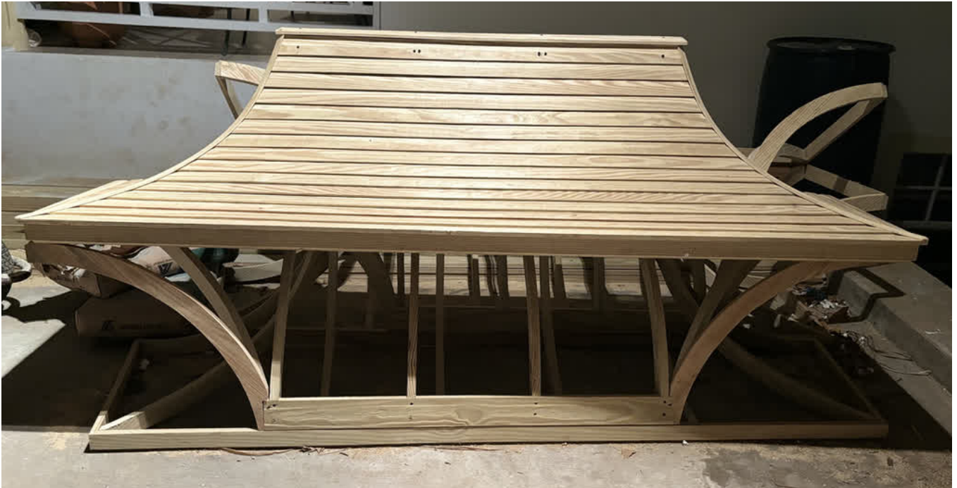
One of the window hoods being crafted for the Codrington House Headquarters.
