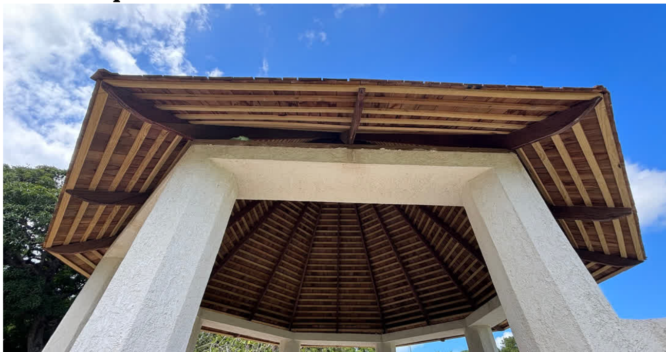
The under view of Trash House's roof
