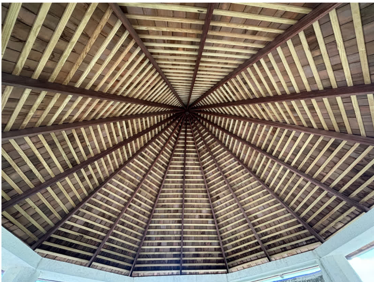
A closer under view of the Trash House's roof
