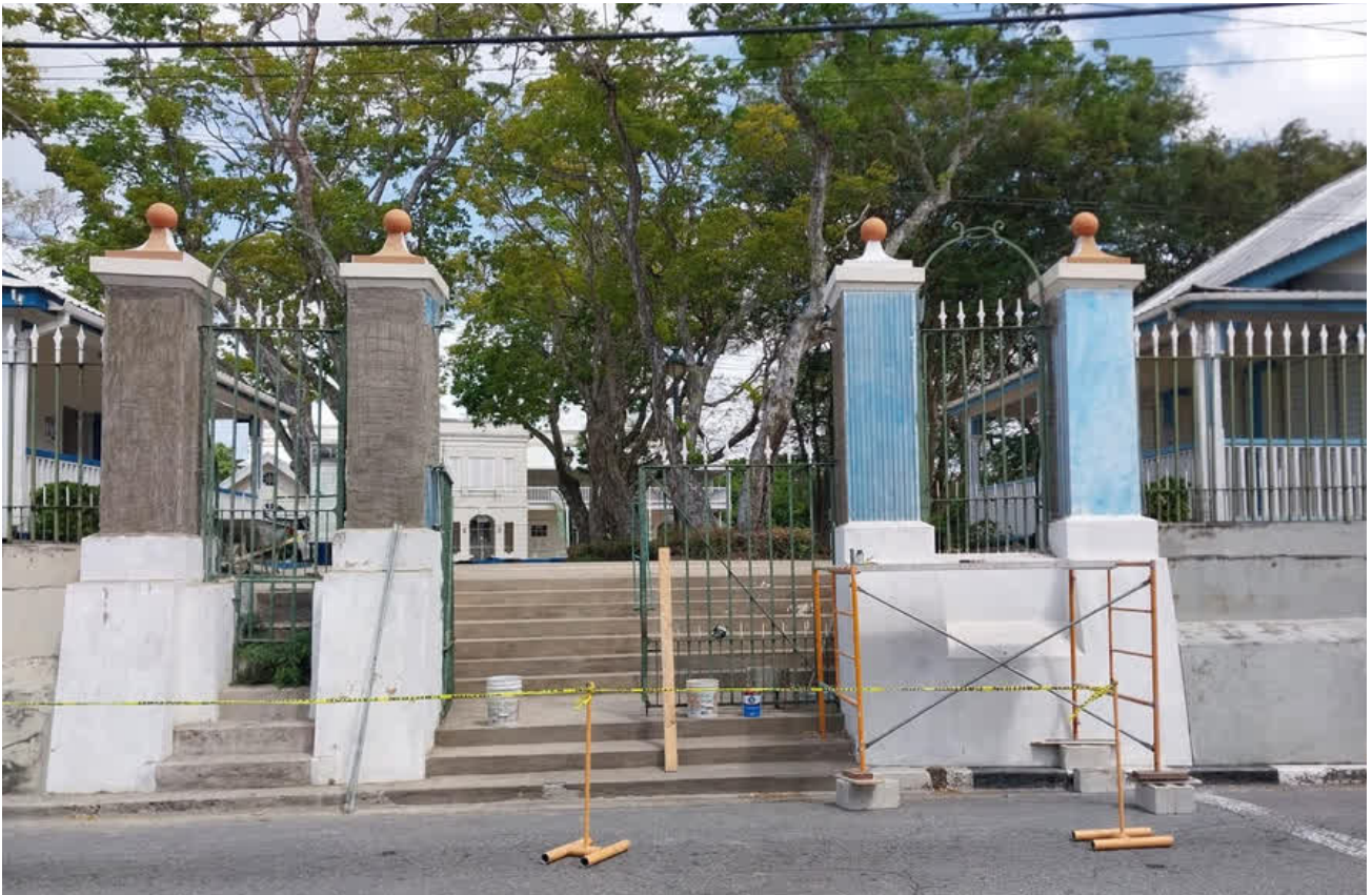
The fiber mesh was covered with mortar after its installation on the columns.
