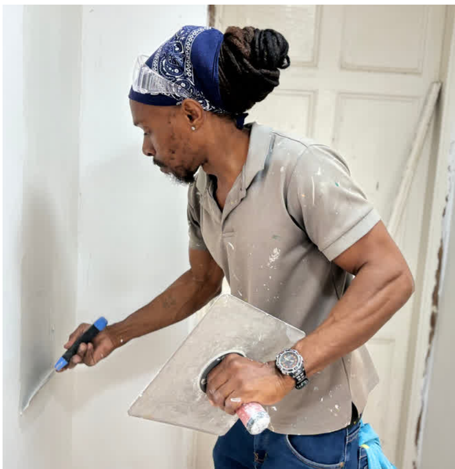
Patrick Hinds applying the slick compound to a wall in the Codrington House’s main office building.
