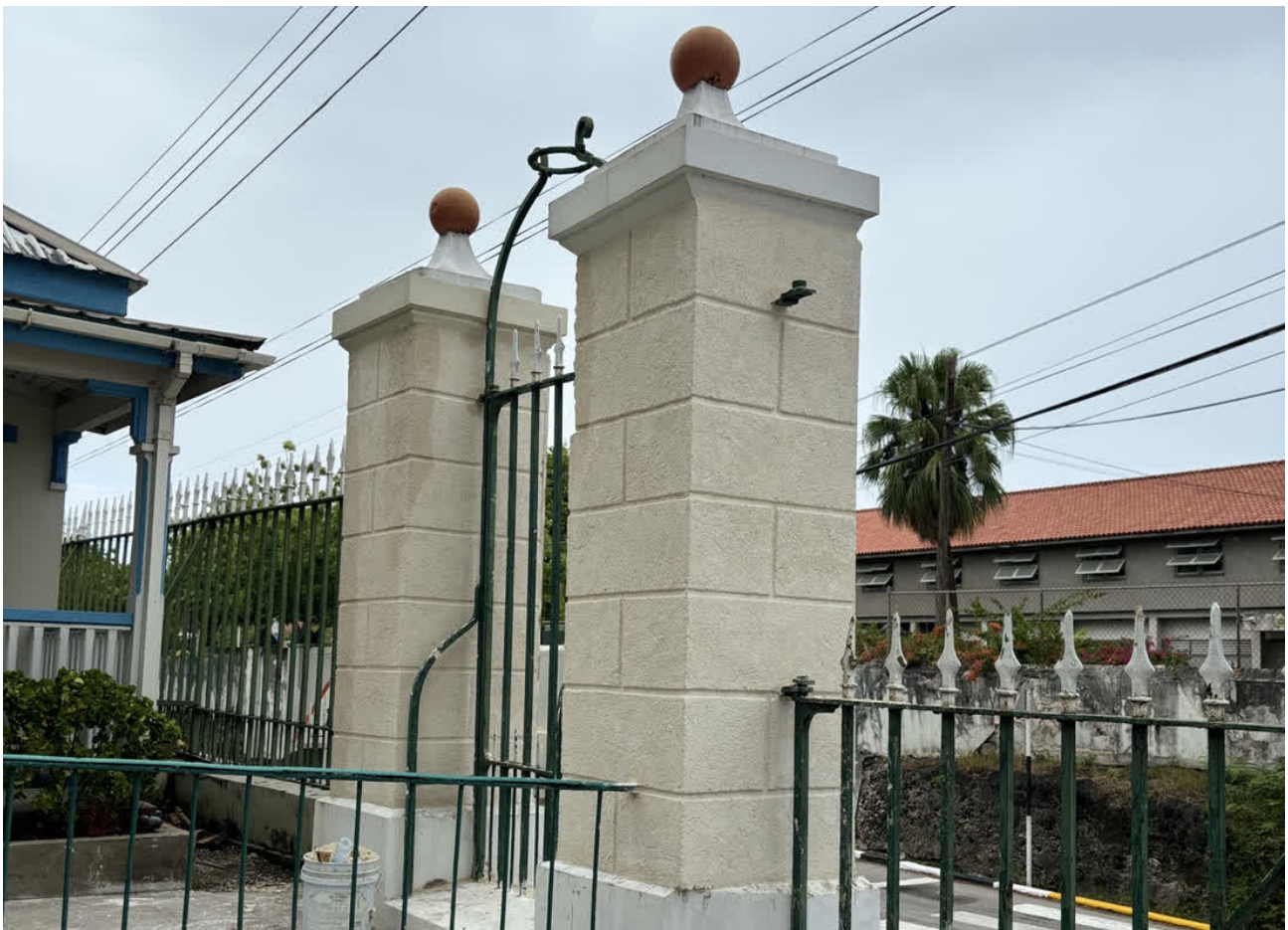
The coral rendered design of the columns before the water glaze was applied.
