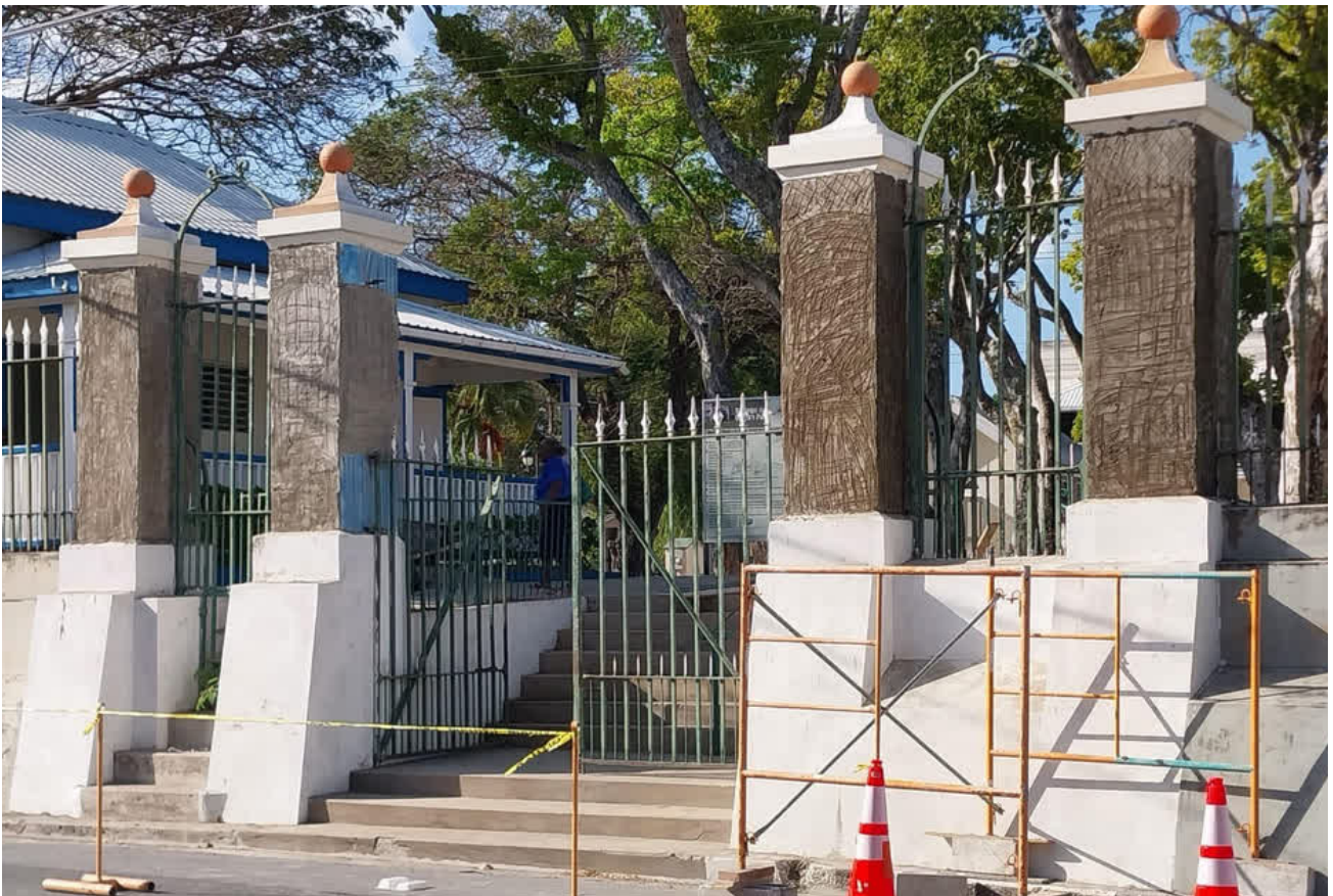
The NCC team also primed the bases of the columns during this phase.
